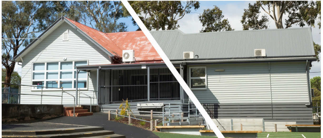
Before and after. The Dulux Acratex team donated paint, equipment and additional funding for skilled tradespeople to work alongside Dulux volunteers as they restored a heritage building, including its ageing roof, at Laburnum Primary School in Melbourne's southeast. The school's 700 students now have a revived Performing Arts Centre.
